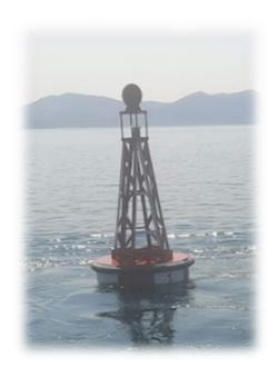
All Aton are on station and fully serviceable. Lights have been changed out and checked to ensure they have sufficient batter capacity throughout the winter.
